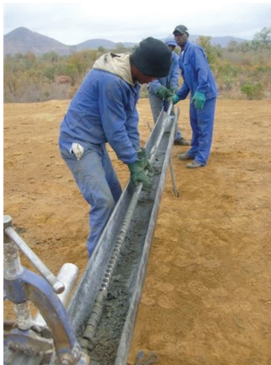
Figure 4. Recovering auger drilled material.
